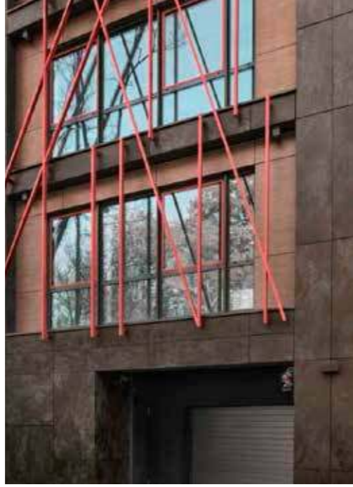
/ Warszawa Year: 2014 Portico Office Building Warszawa /Poland Laminam 3+ Ventilated Facades Oxide Nero 1000x3000 >
