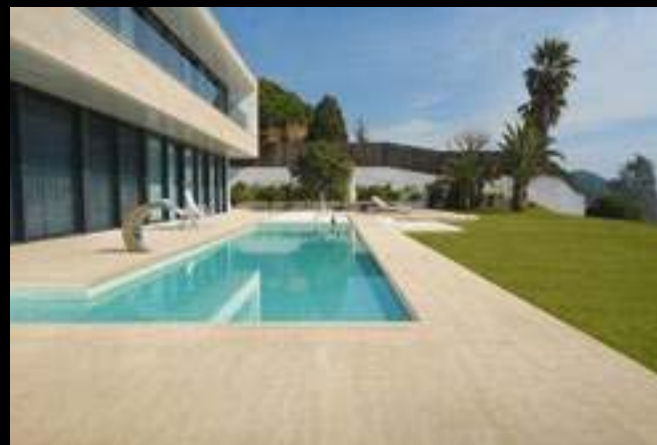
Pool Villa - Sand Vein Cut & Cross Cut
